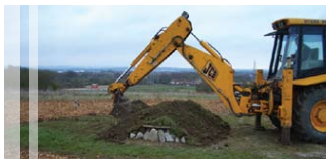
Reptile and GCN hibernacula construction
